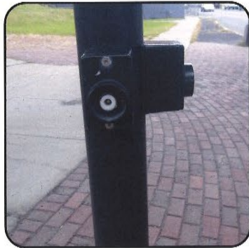
Intersection #1 Hoosick Street/River Street
