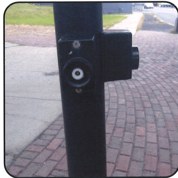
Intersection #1 Hoosick Street/River Street
