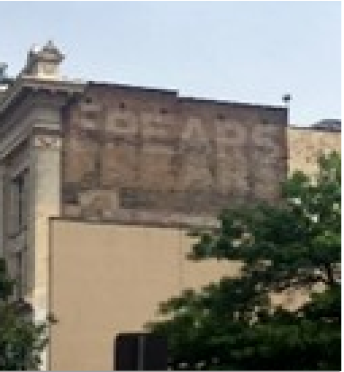
Historic signage is to be preserved, and restored whenever it is possible
