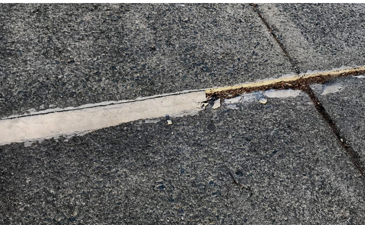
Concrete filler can be used to level uneven surfaces but it won't last long
