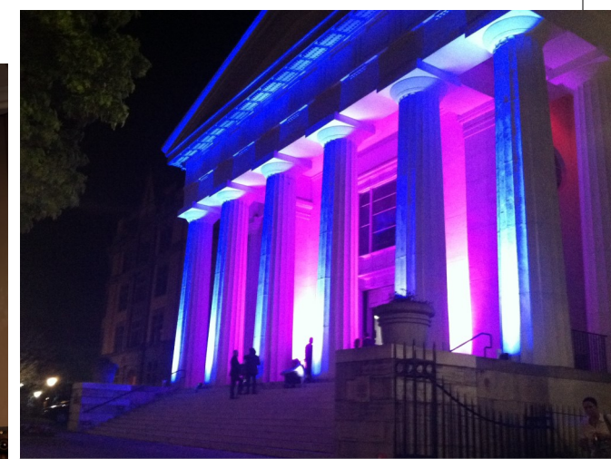
Advances in lighting technology make dramatic artistic lighting possible.
