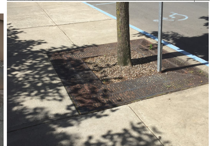
Tree grates must be no more than 1/2" out of level with the surrounding sidewalks.
