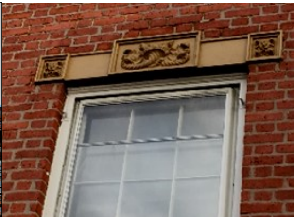
Pressed metal and cast building component were cost cutting measures 100 years ago. Ironically they have lasted far longer than their sandstone counterparts may have.
