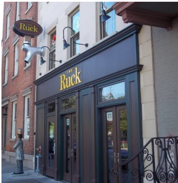
The completed project restored a pub type façade and corrected the poor window choices above. Creative signage was also installed.
