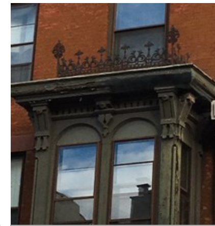
Cast iron cresting is rare now and should be preserved with a good coat of paint
