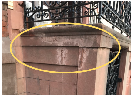
As with brick masonry, inappropriate sandstone patches are easy to spot
