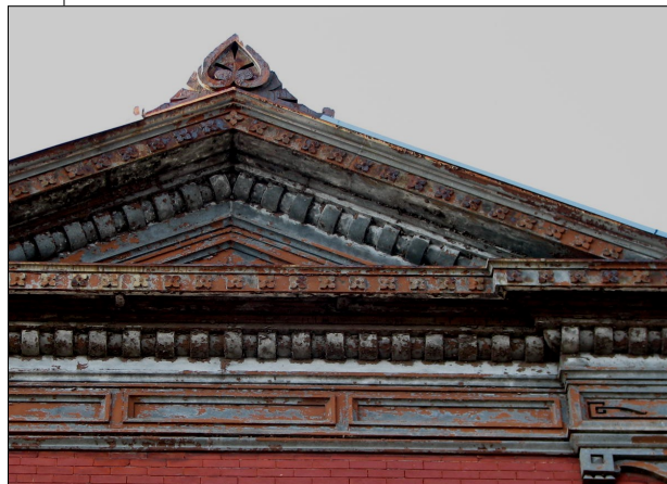
Pressed metal and cast building component were cost cutting measures 100 years ago. Ironically they have lasted far longer than their sandstone counterparts may have.
