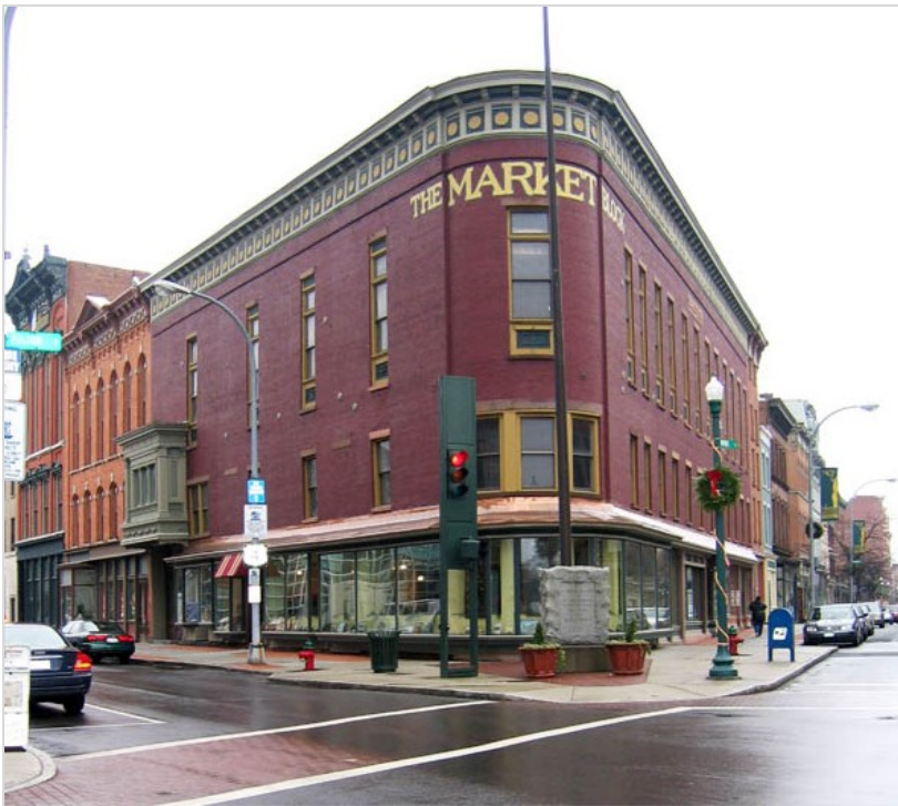
The Market Block, at River and Third Streets, is a collection of six buildings renovated to share an elevator and a common circulation and service core. Creative solutions like this allow older structures to comply with current building codes.
