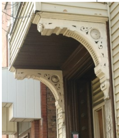
Vinyl covers all but 2 brackets on this house
