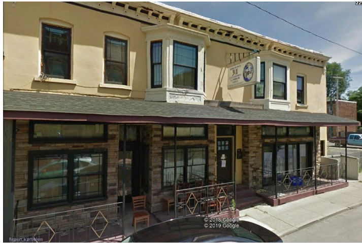
This inappropriate porch was added where none existed. The same effect could have been achieved for less expense with awnings and street furniture.
