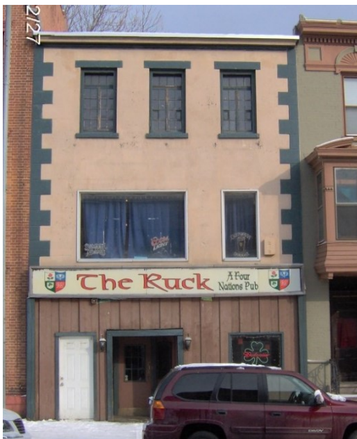
An inappropriate 1970’s renovation interrupted the window rhythm and fortified the traditional storefront.
