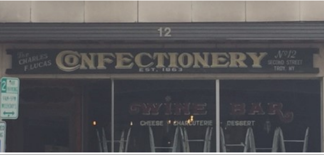
The band of space between the storefront cornice and the glass is traditionally used for signage. Add light fixtures directed on the band for best effect
