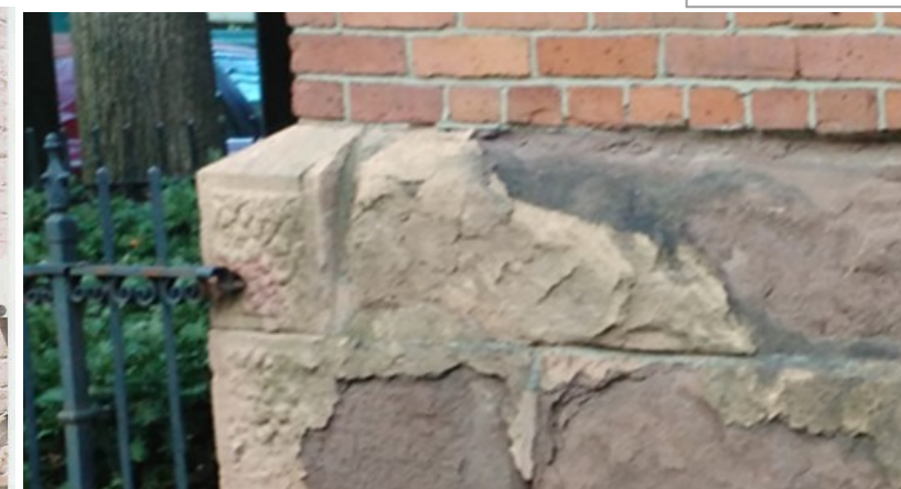
Stone building components that are beyond repair can be replaced with more durable materials, such as cast stone, glass fiber reinforced concrete and, in rare occasions, a resin component may be used.
