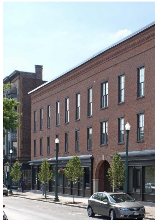
The Chazan Building renovation restored an arched entry on Broadway that had been hidden by earlier inappropriate work.
