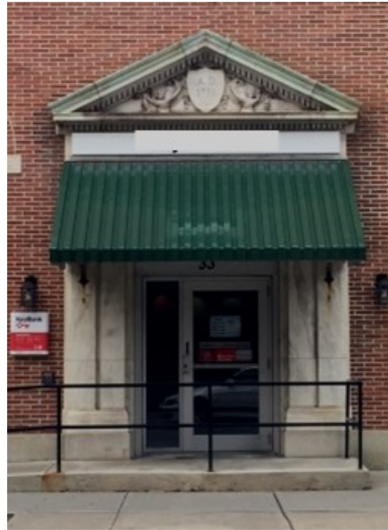
Contemporary metal awnings are not appropriate and this awning obscures the architec-
