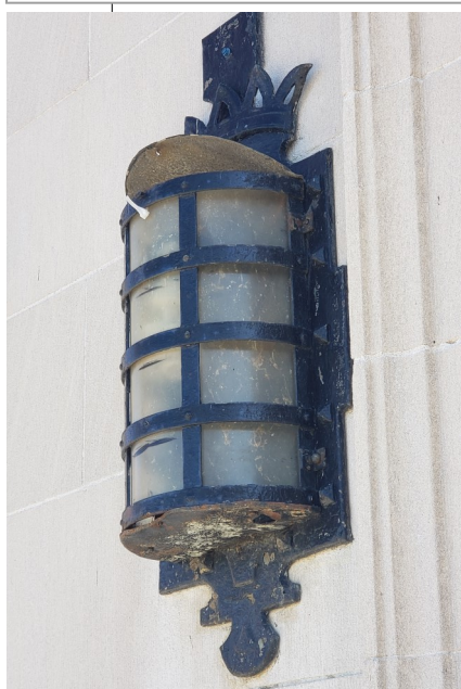
Historic fixtures can be restored and fitted with new LED technology. If maintained well they will last another 100years. Electrical wiring should be done by professionals. There are lighting supply companies in the region who do this very well.
