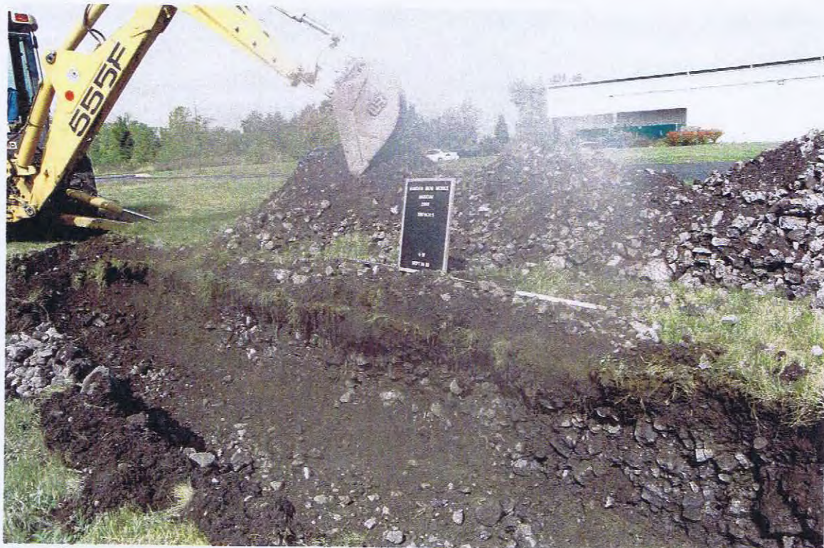
5. View northwest of the north wall profile of Trench 3 showing three levels of fill on top of a solid slag surface.
