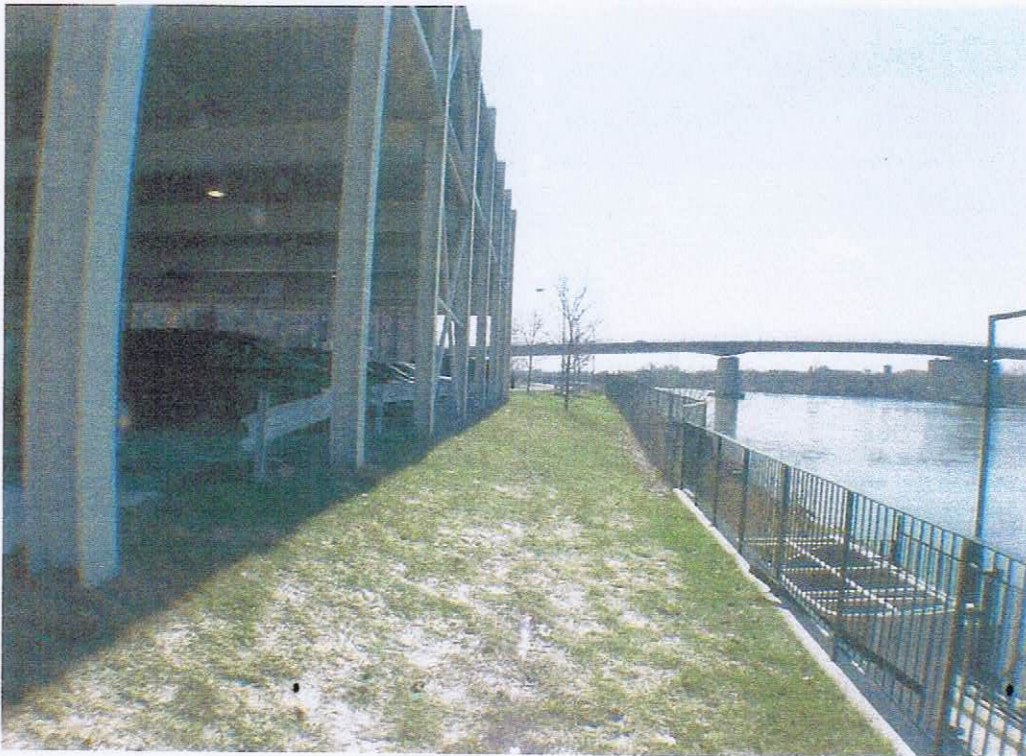
23. View southwest. The trail will be located along the grassy area.
