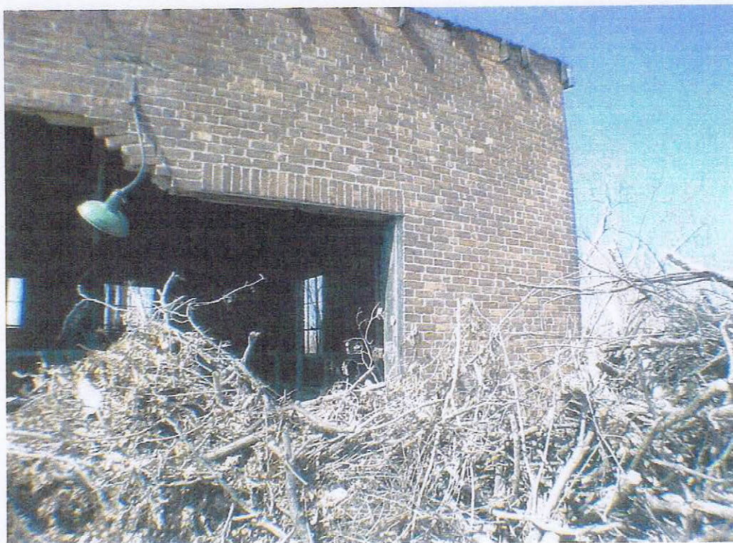
6. View northwest of the brick pumping station.
