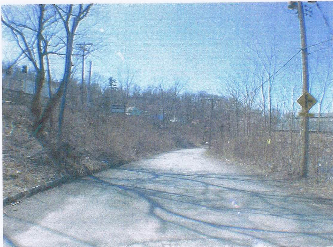
2. View south near the southern terminus of the project area. The trail will be placed along the left side of the road here.
