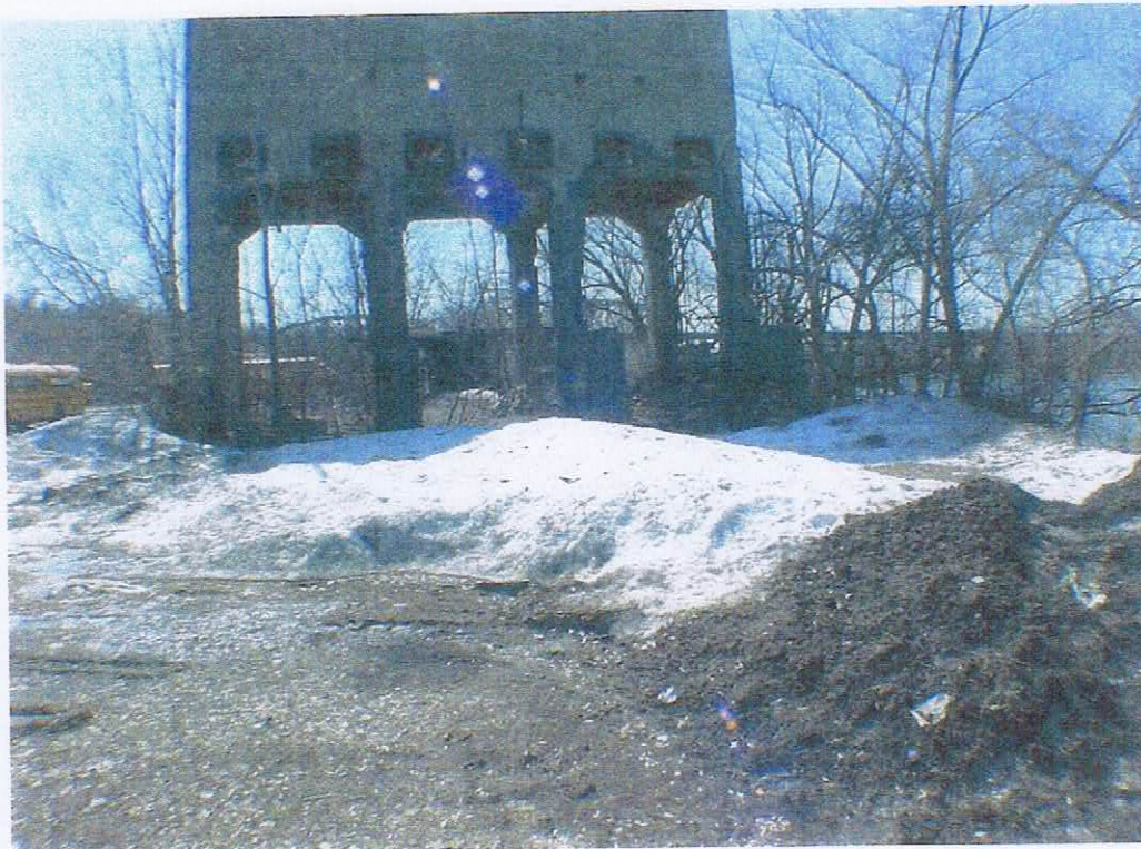
5. View south. The poured concrete silos in the foreground and a cinder block workshop/garage beyond the silos will be demolished for the project.
