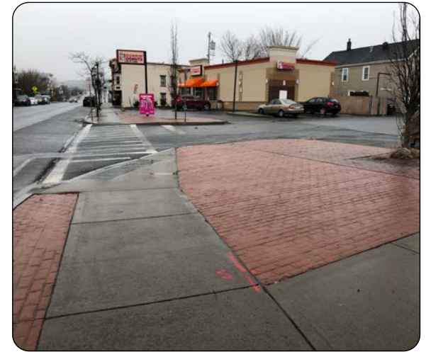
Photo 5: Stamped asphalt at 4th Avenue intersection bump-out.
