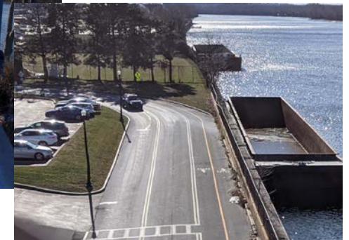
Front Street cycle track - view from bridge
