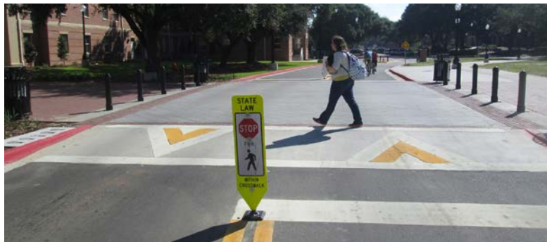
Wide raised crosswalk on the USM campus
