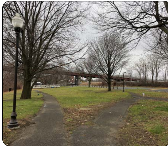
Photo 2: Asphalt pedestrian path continues toward bridge.
