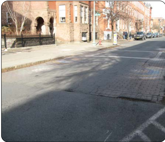
Photo 6: Pedestrian crosswalk on 1st Street. Stamped asphalt in poor condition. Decorative paint is mostly worn away.
