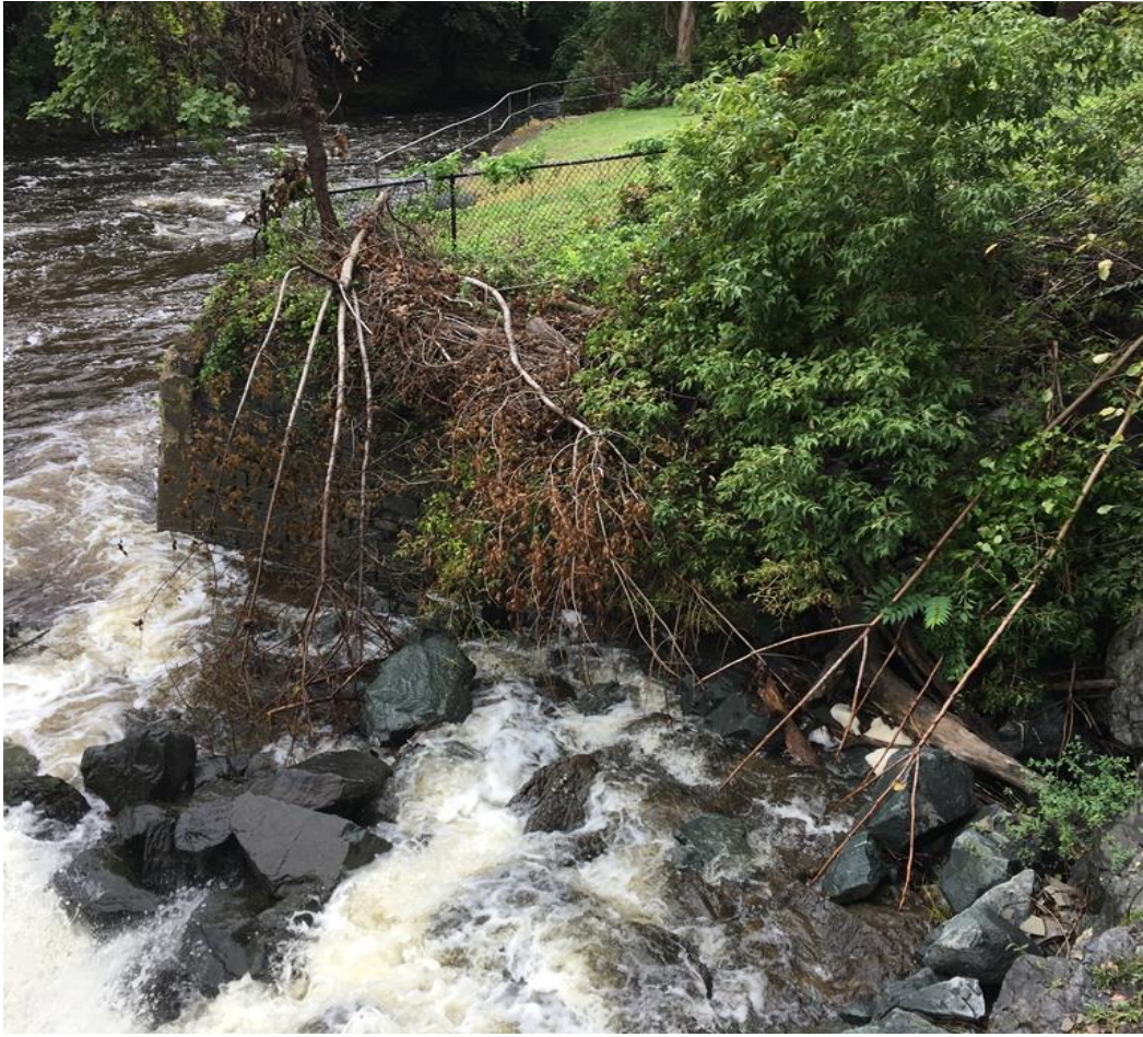
Photo 4 Dam ID# 226-1391 Ida Lake Dam 09/28/2018 Right downstream wing wall
