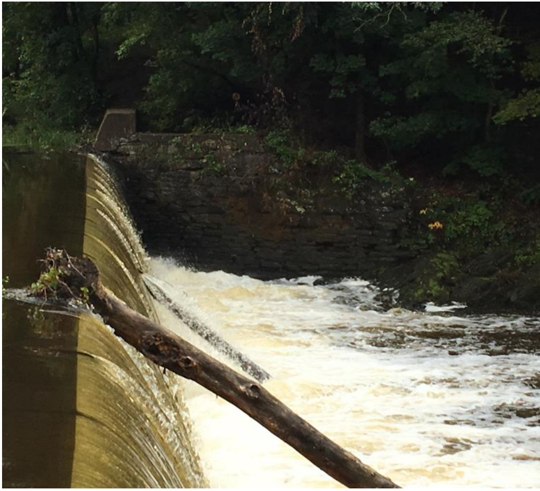
Photo 2 Dam ID# 226-1391 Ida Lake Dam 09/28/2018 Left abutment wall
