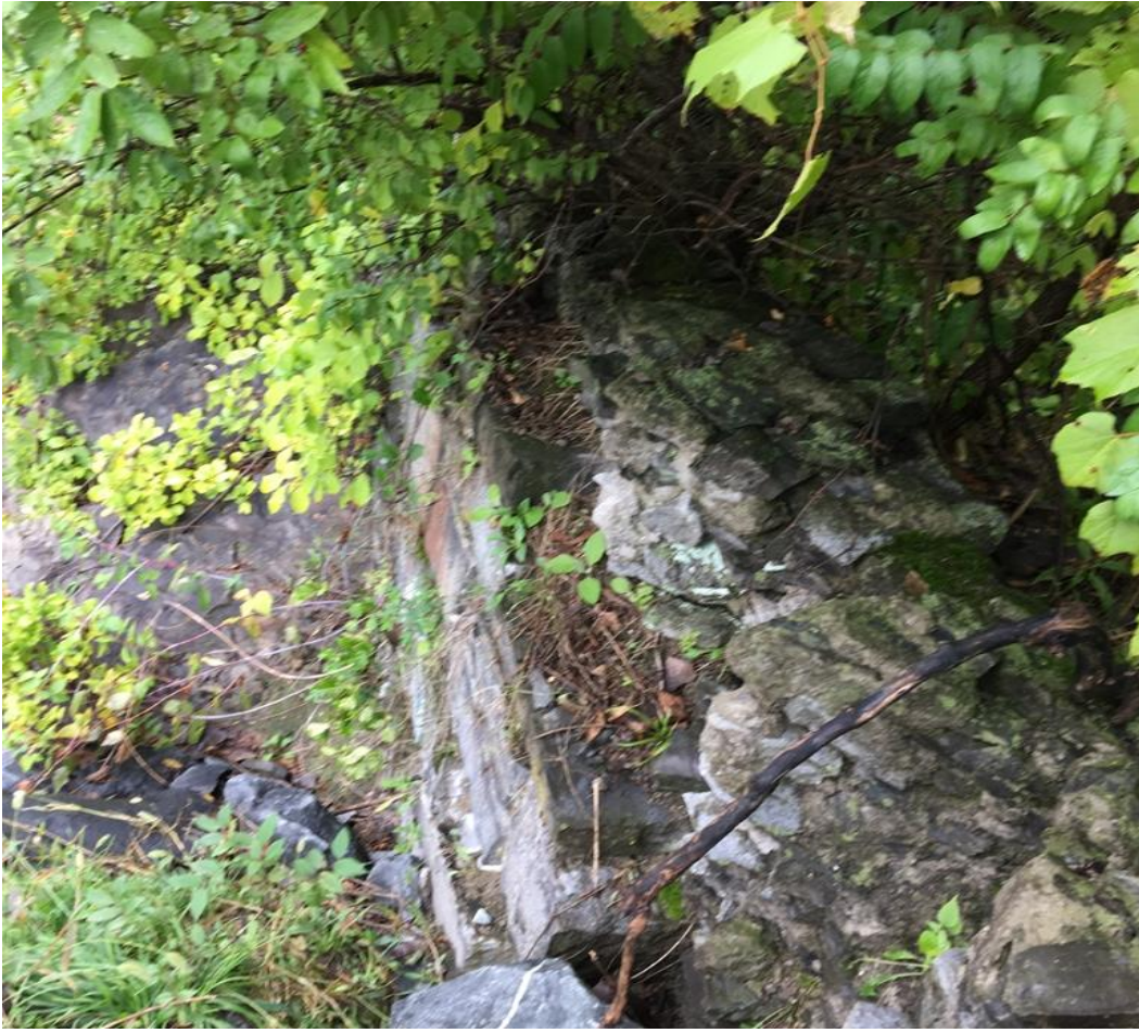
Photo 3 Dam ID# 226-1391 Ida Lake Dam 09/28/2018 Right downstream abutment wall looking downstream
